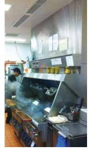
Above left: An alternative arrangement is to supply Climate Wizard air directly above the cooking appliances to provide a "curtain" of cool air that is extracted by the range hoods.
