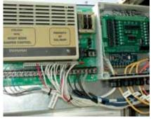
Above: In order to fully integrate the economiser (outside air cooling by Climate Wizard with the normal RTU function) a PLC was employed with dictated system response to climatic conditions and the indoor heat load.
